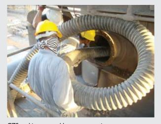
CZS packing removal by vacuum car in progress
