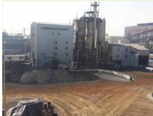
By-Products Briquetting Plant
