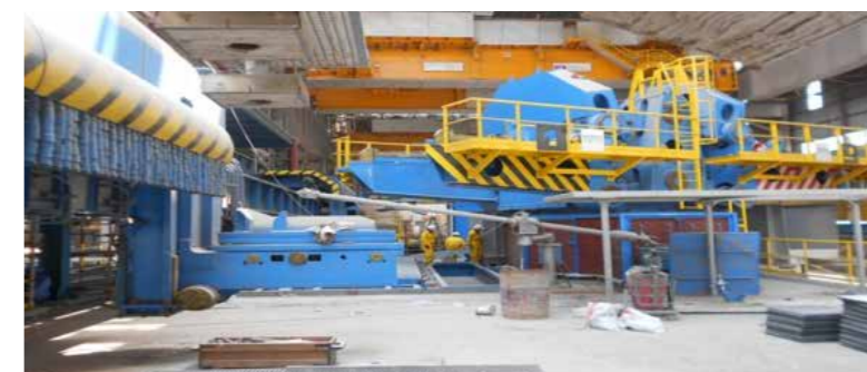
(CCM's casting platform-Ready for Refractory work)
