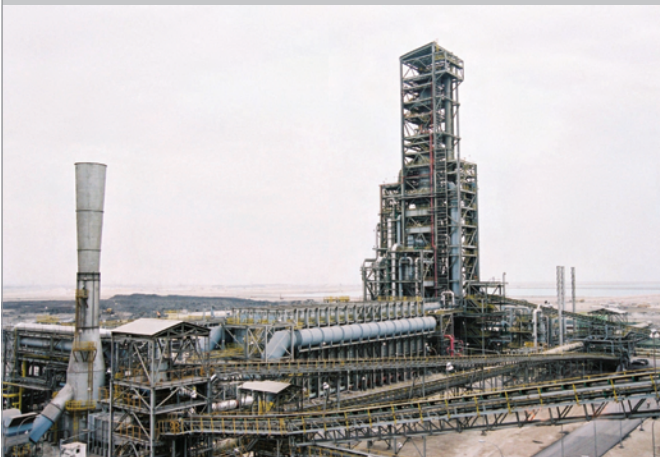
View of the core plant area
