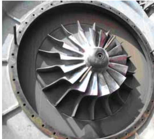
New Impeller Installed in the First Stage Process Gas Compressor in DR-2 (April 2009)
