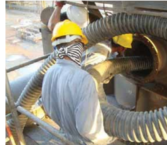
Scrubber Packing Removal by Vacuum Car in Progress in DR-1 (May 2009)
